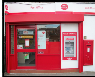
Horden Post Office undergoes Refurbishment
