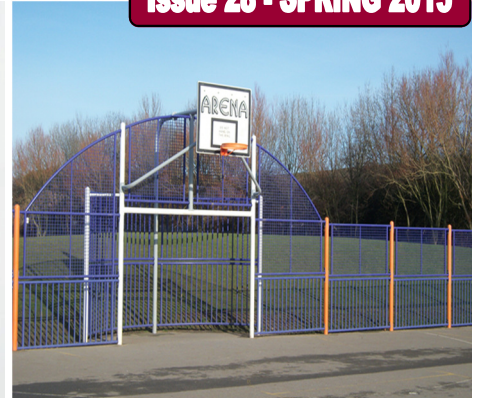
Details of the future of the Staplyton Drive MUGA inside
